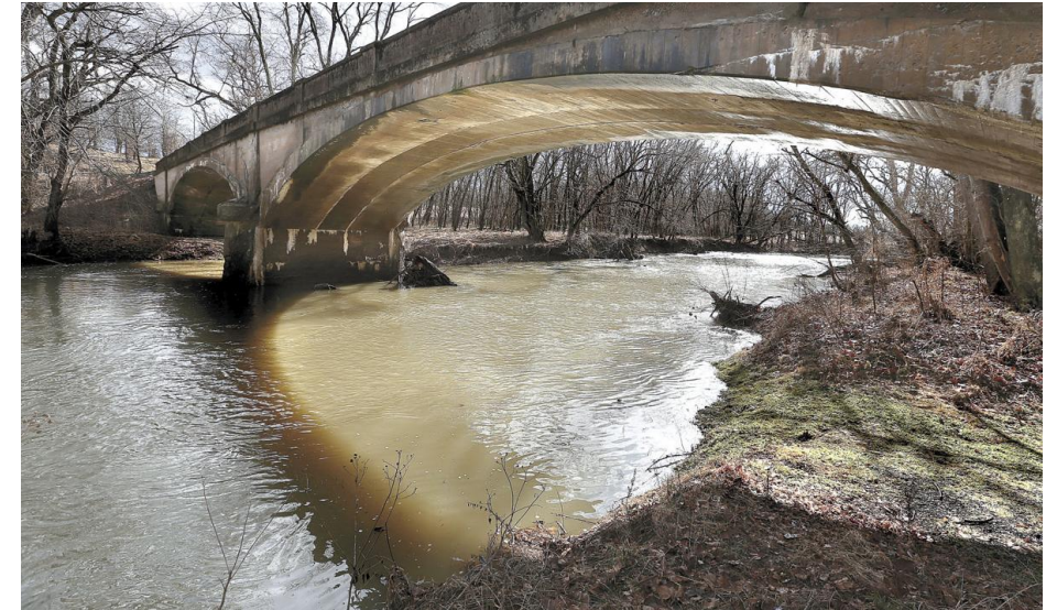
Opequon Creek, Frederick County, VA, USA Source: Winchester Star, Jan 23, 2018 ( link )
