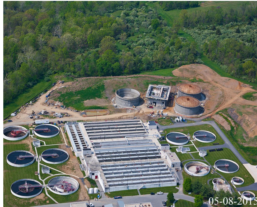
Opequon Wastewater Treatment Plant, Frederick County Sanitation Authority, Winchester VA, USA
